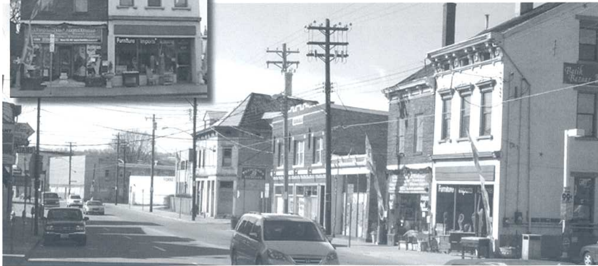
Lack of physical access to Spring Grove Avenue merchants has dampened business and caused safety issues.
