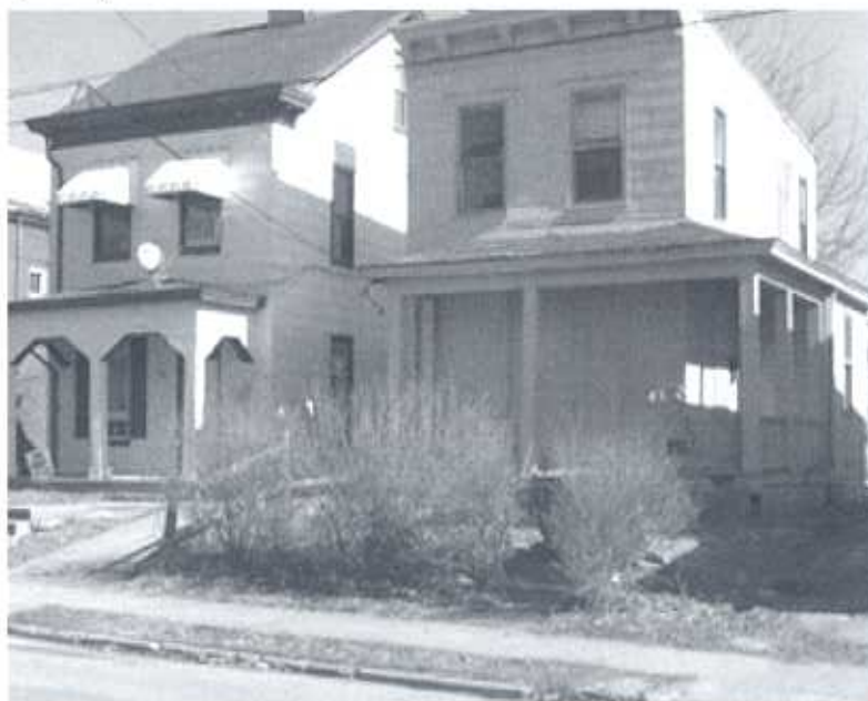
Poor housing conditions on Fergus St.
